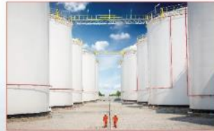
Successful commissioning and start-up of phases 1A and 1B
