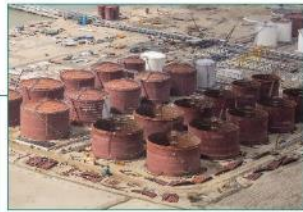
Construction of tank terminal in three phases: 1A (432,000 cubic meters) 1B (432,000 cubic meters) 1C (420,000 cubic meters)
