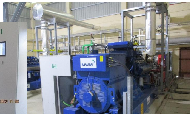
Typical Type of Biogas Engine for Power Generation
