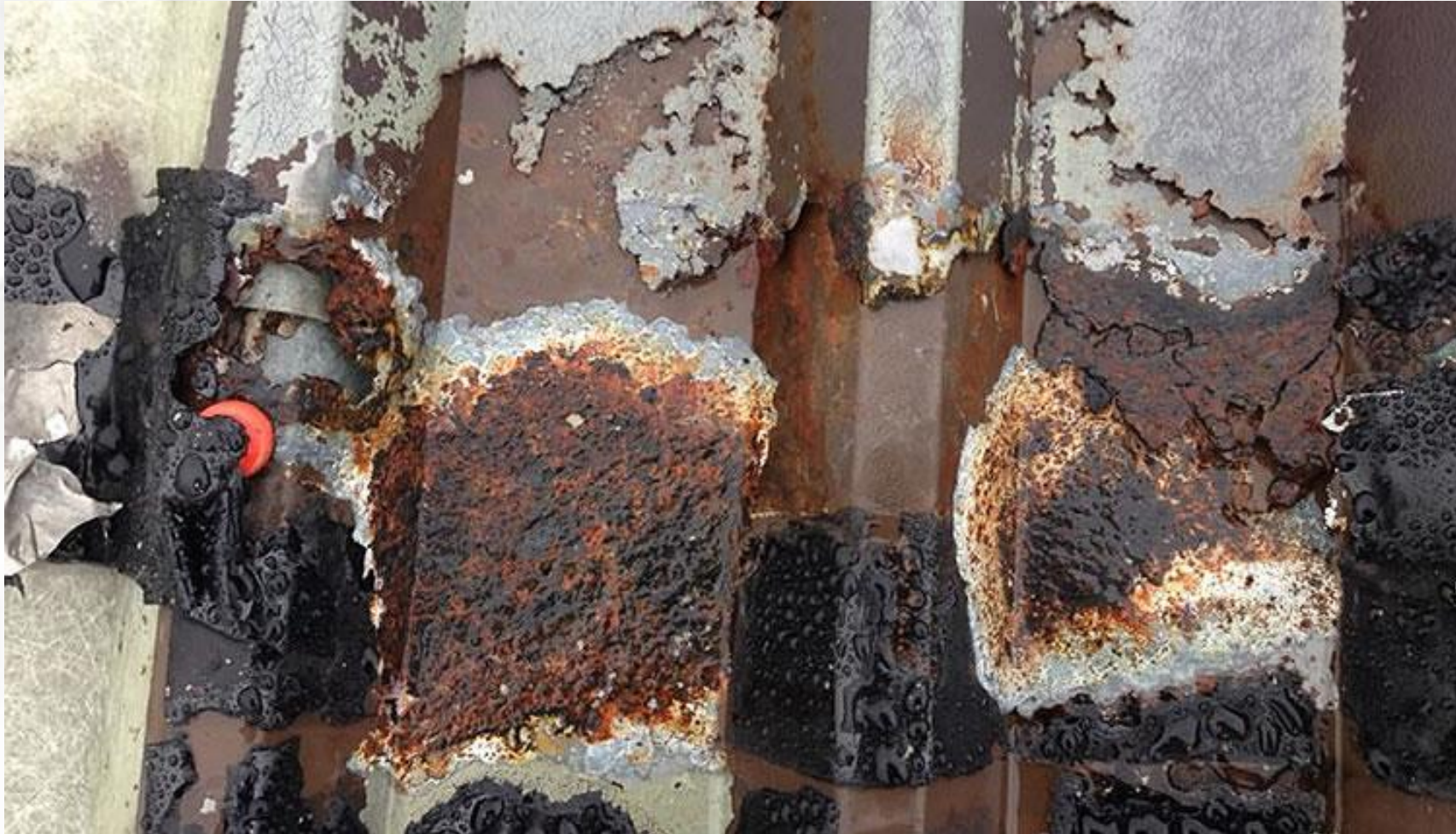
Corrosion under paint
