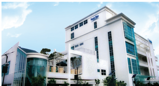
Basis Bay - Builders of Asia's First Green Data Centre
